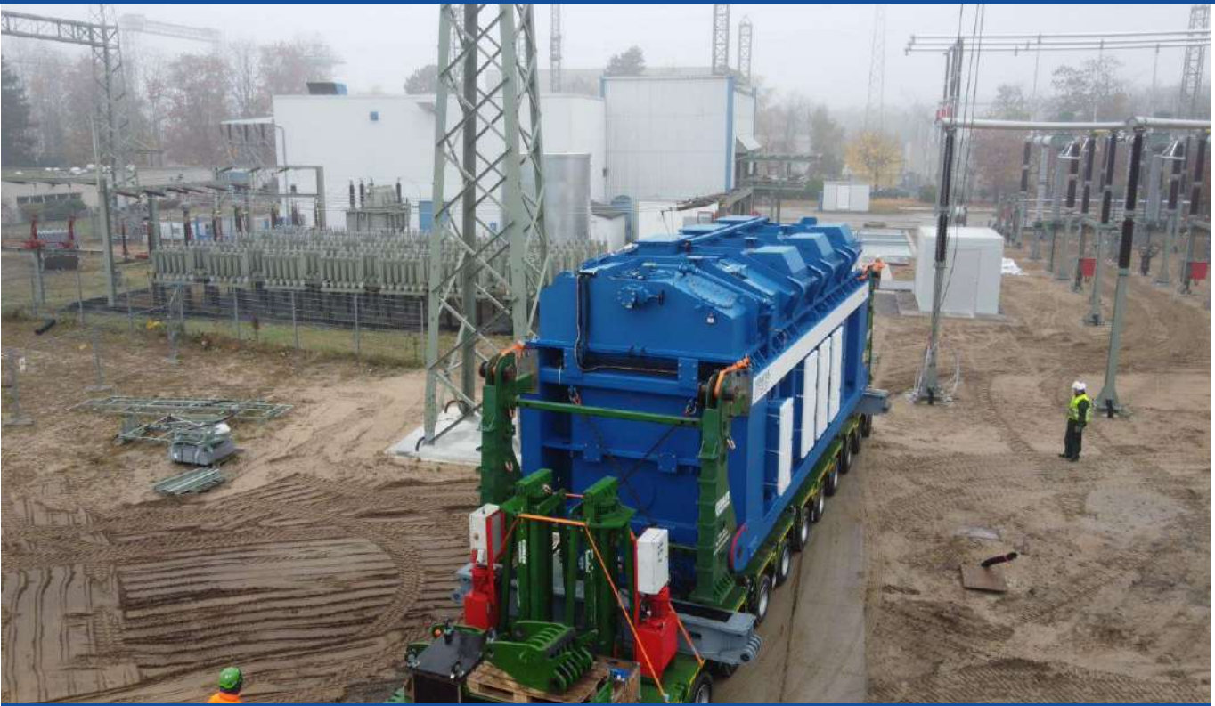
Installation of Transformer T401, built by Siemens Energy, at KEMA Labs in Mannheim (Germany)
